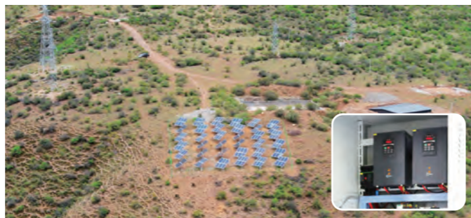
95kW Controllers: 2*PDS33-4T037 Location: Sichuan Province, China
