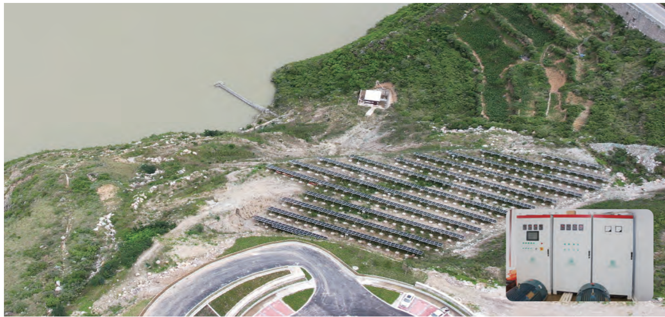
315kW Controllers: 4*PDS33-4T075 + 4*PDS33-4T18R5 Location: Sichuan Province, China
